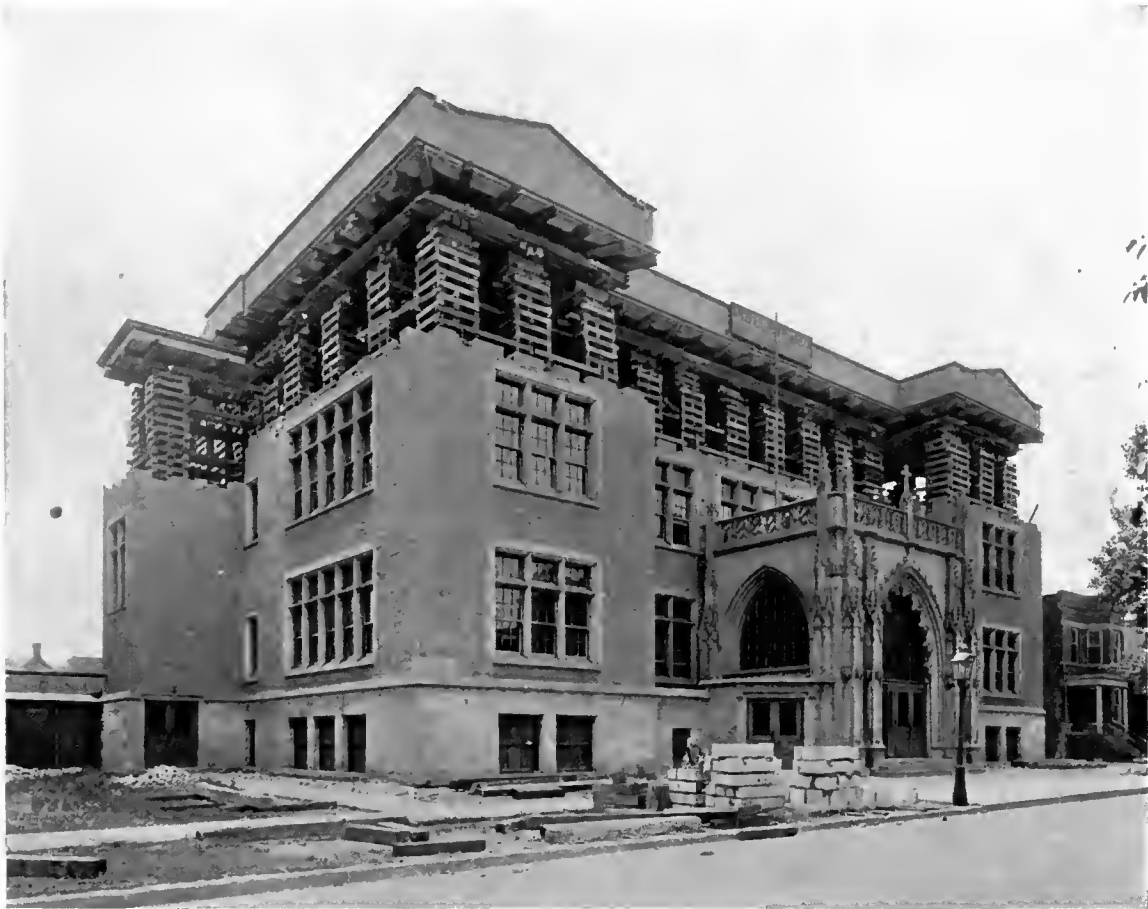
VIEW SHOWING ROOF RAISED AND SUPPORTED
